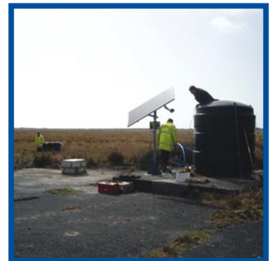
Installation of the pump and water tank.
