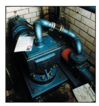
Public toilets, located directly beneath a local tourist information centre, are open 24 hours, but not attended at night. This results in abuse of the drainage system, with drink cans and other items of indiscriminately disposed of waste found in the sump. A compressed air operated sewage ejector system was previously installed but could not cope with this abuse. It required weekly maintenance visits and was extremely noisy.
