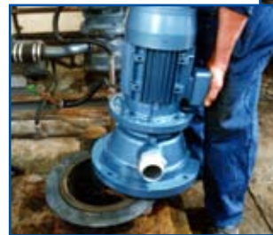
It is easy to retrofit an M18 macerator!
